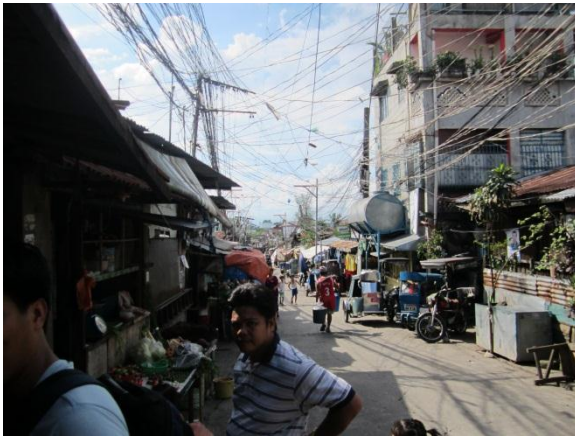
Danger zone under the high voltage electric wire
